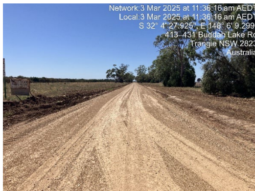
Figure 1: Recent grading and gravel resheet on Buddah Lake Road (left) and Ceres Siding Road (right)
